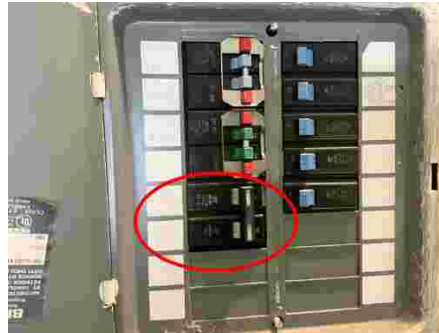
40 amp fuses exceeds max per label
