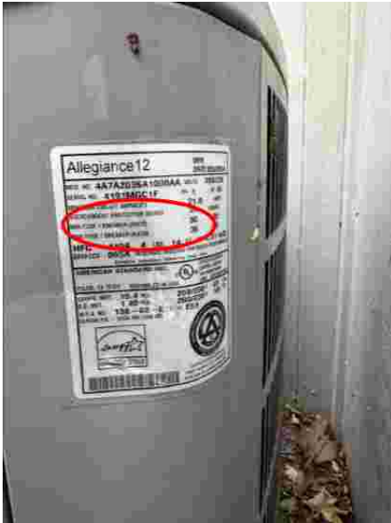
40 amp fuses exceeds max per label
